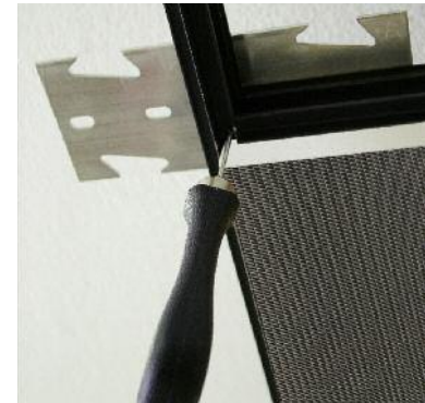
Rotate hook behind panel.
