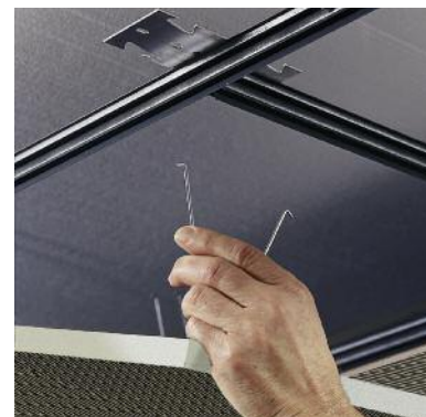
Disengage panel retainer springs from "butterflies".
