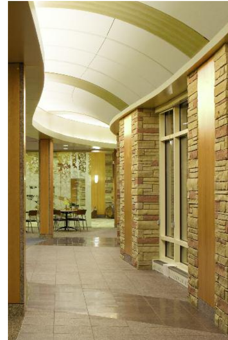
Curved custom Ceilencio ceiling with Claro and Quadrillo panels enhance the vaulted corridor of this medical centre lobby.
