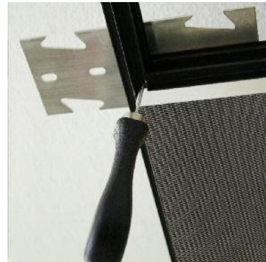
Rotate hook behind panel.
